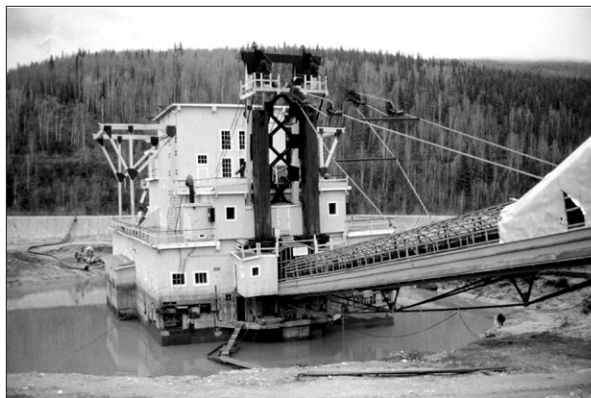
Relocation of Dredge No. 4 NHSC
