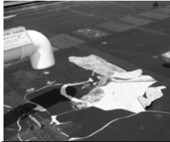
courtesy of Performance of Roof Systems & Insulation, Institute for Research in Construction
