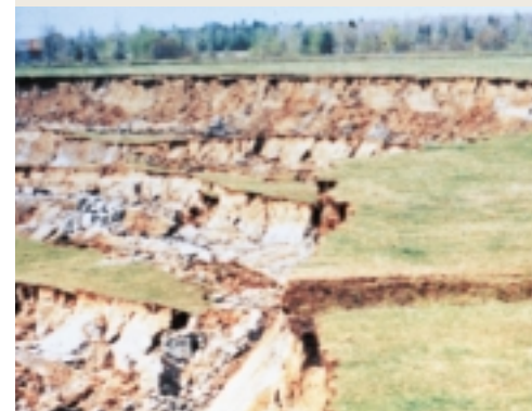
Massive slope failure
