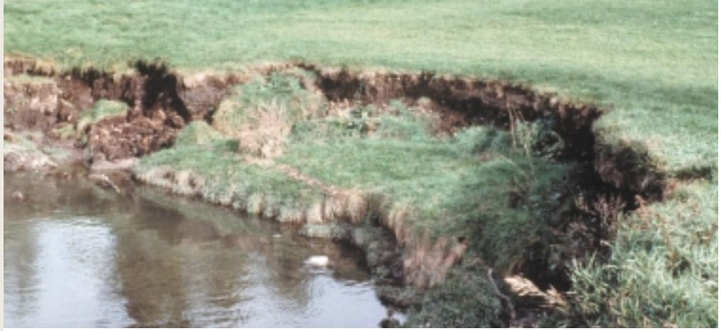
River bank erosion
