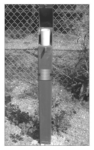
Clamp the tag around the casing with a stainless steel strap or, if strapping is not possible, tac weld it into place with stainless steel rods.
