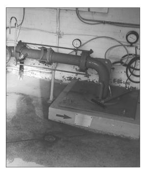
The presence of a well house does not affect the placement of the well tag. The tag location depends on whether the pump is positioned directly over or offset from the casing. Follow the directions in Scenario #1 or #2, whichever is appropriate. In addition, the well owner is encouraged to post a sign on the outside of the pump house, either next to the door or on the door, indicating the well tag number.
