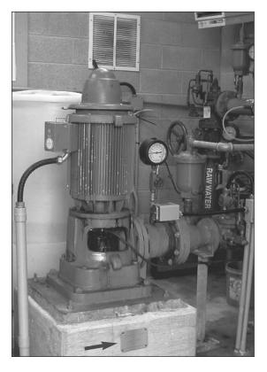
This scenario would include wells with a vertical turbine pump, hand pump or other type of pump positioned directly over the casing. Set or lag the well tag into the concrete well slab as close to the casing as possible, while ensuring the tag remains visible and protected from undue wear and tear.
