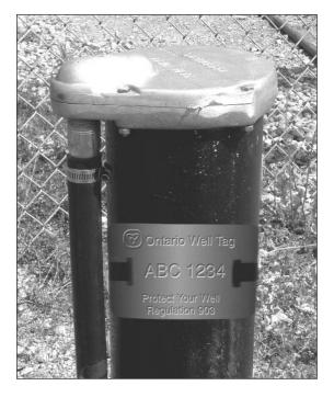
This scenario would include wells with a submersible jet pump, suction pump or similar pump. Clamp the tag around the casing with a stainless steel strap or, if strapping is not possible, tac weld it into place with stainless steel rods.
