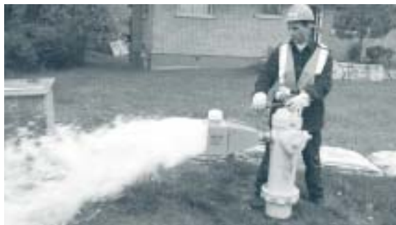
Municipal operator flushing and checking flow of distribution main
