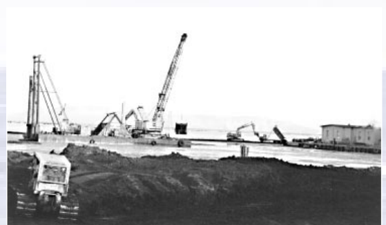
Removing polluted sediment.
