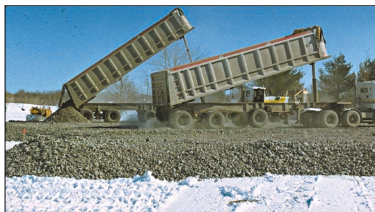
Covering the red mud tailings with crushed limestone.
