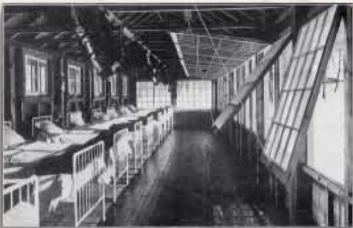
Interior view of Kendall Pavilion of the Muskoka Cottage Sanatorium, showing arrangement of glass front. Illustration from The Muskoka Cottage Sanatorium [pamphlet], [ca. 1928]. (National Sanitarium Association fonds, F 1369-2-0-2) MU 2772
