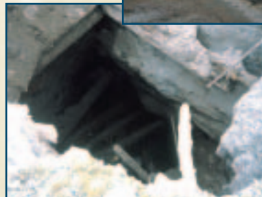
◀ Abandoned mine shaft before it was sealed
