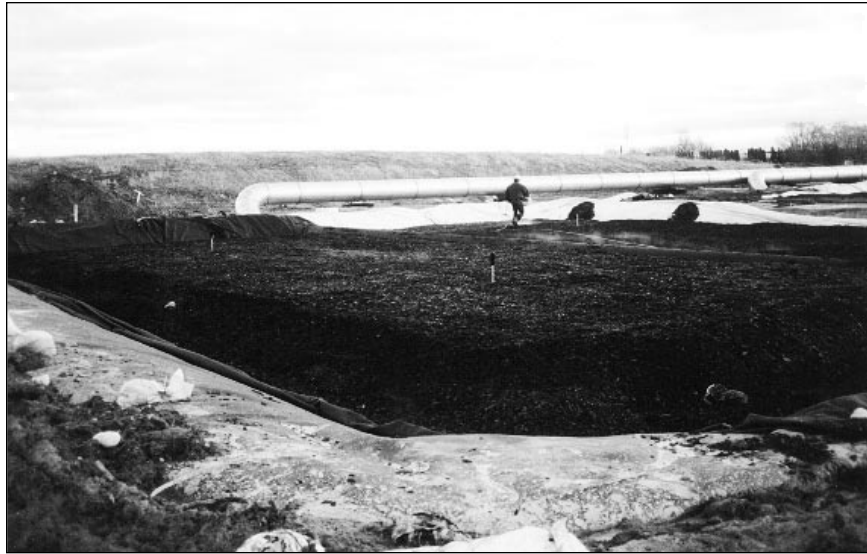
Biological air filters at Maple Lodge Farms have proved to be very effective in eliminating odour.
