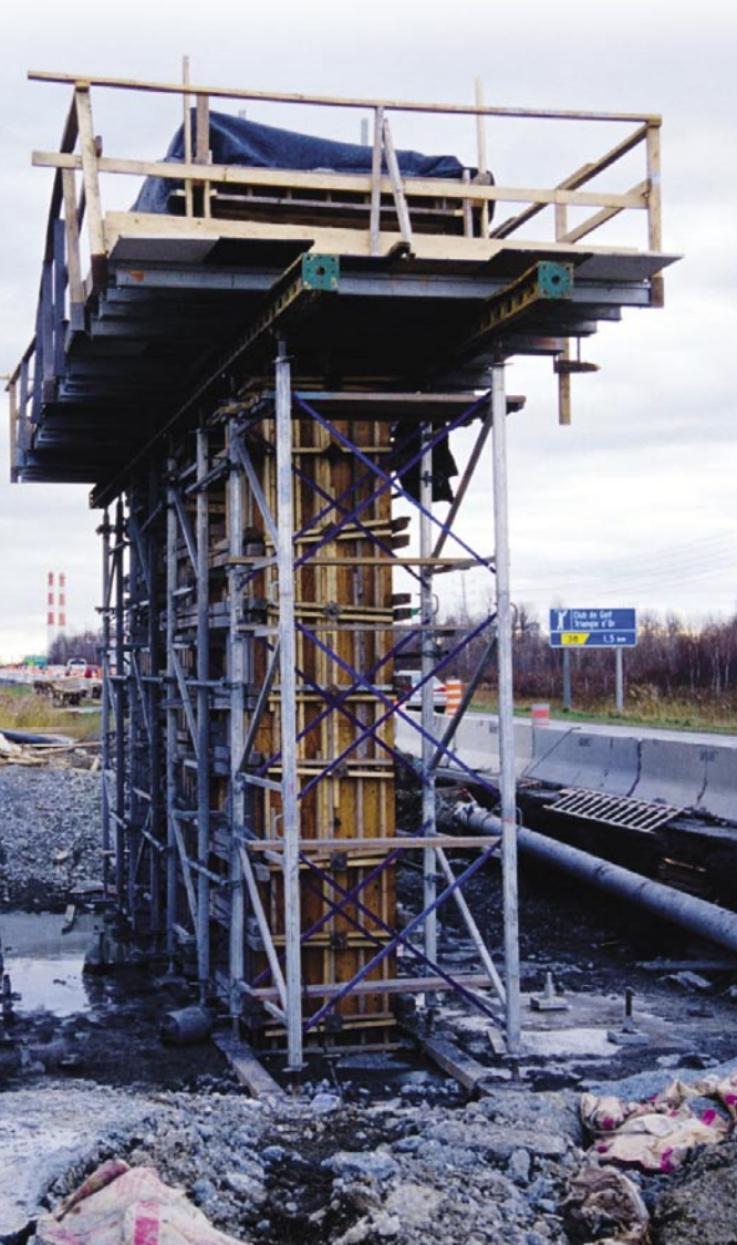
Work on the overpass started during the summer of 2005.
