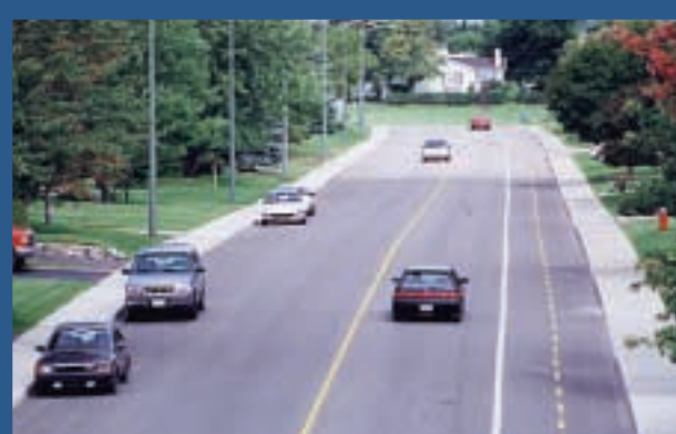
Here, the width of the paved surface includes the two traffic lanes, a parking lane and a bicycle lane.
