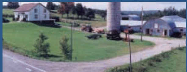
Main access point for farm with buildings
