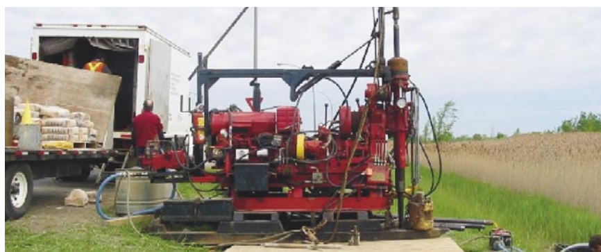
Equipment used for this type of drilling in quick clay.
