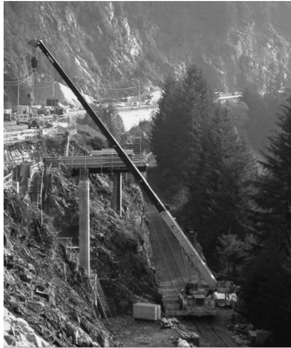
Construction north of Horseshoe Bay
