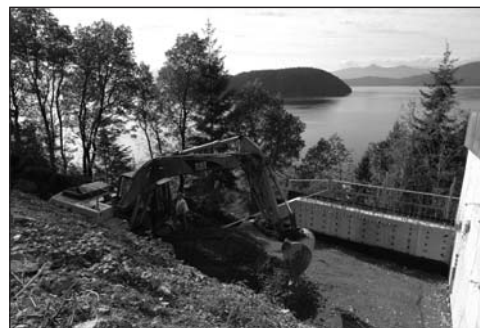
STS Hwy — Building Retaining Wall
