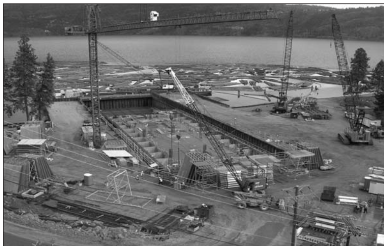
William R. Bennett Bridge Installation of Top Slab Formwork.
