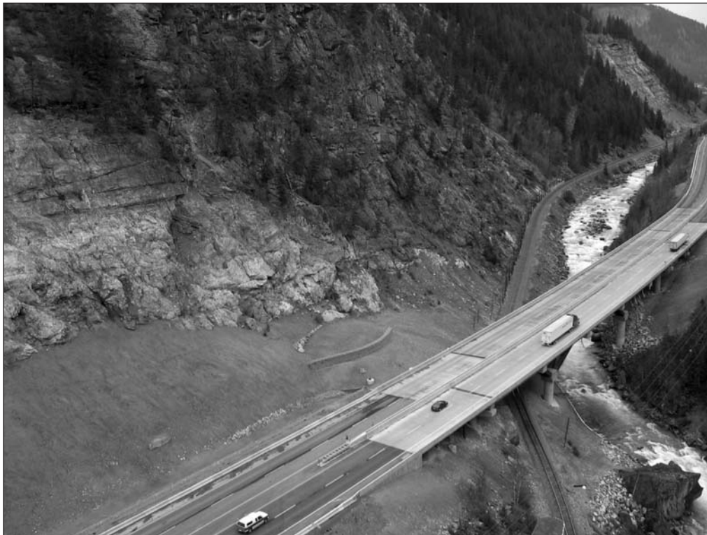
Kicking Horse Canyon New Yoho (5-Mile) Bridge
