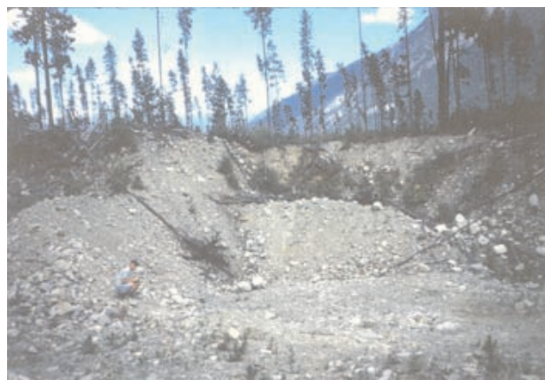
Figure 3. Typical borrow pit used to facilitate logging road construction. Pits are generally small (~2000m 3 ) and exploit local material to reduce transportation distance (forest service road south of Birkenhead Lake).
