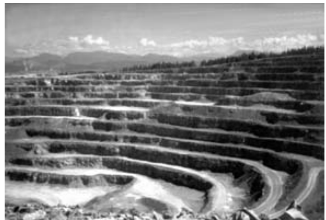
Photo 5. A photo of the main pit at the Blubber Bay Quarry; a limestone quarry located on Texada Island. This pit is approximately 160 m deep.
