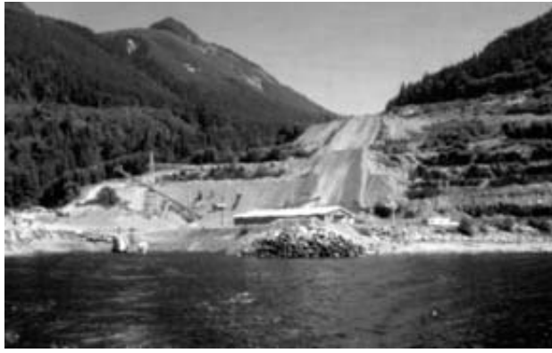
Photo 2. A medium to large-scale aggregate pit located on Jervis Inlet called the Treat Creek Pit (Jack Cewe Ltd.).
