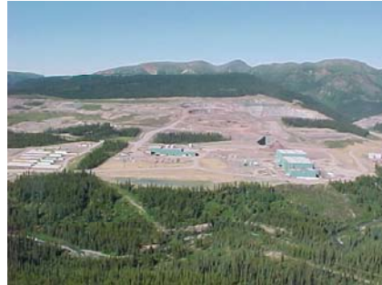
Figure D-1 Northgate Minerals, Kemess Mine
