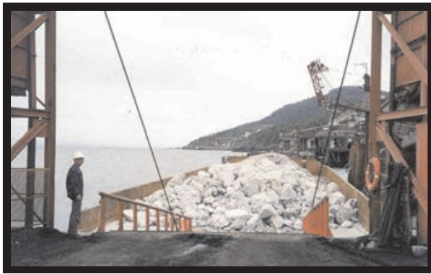
Figure 7. Gillies Bay Loading Facility, Vancouver Island; Texada Quarrying Ltd.
