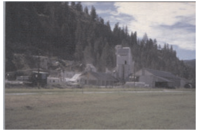
Figure 8. Dolomite processing plant near Rock Creek; Mighty White Dolomite Ltd.
