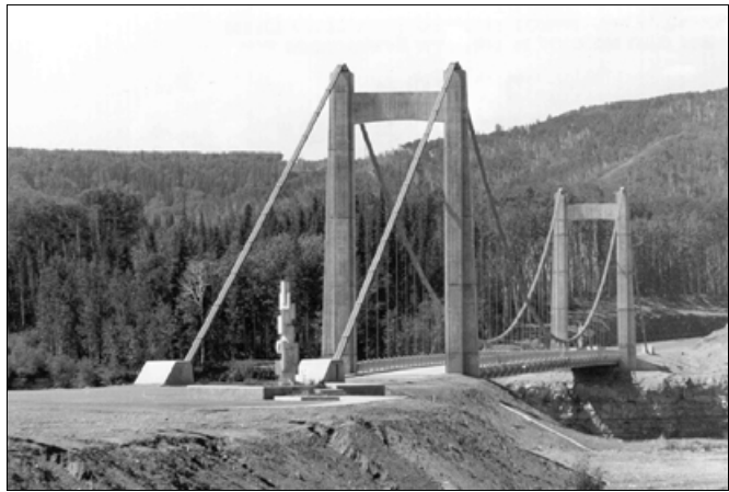
Peace River Bridge on Highway 29 near Hudson's Hope.
