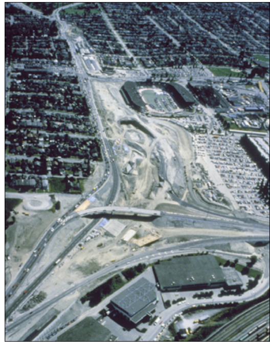
(Above) Cassiar Connector, under construction.
