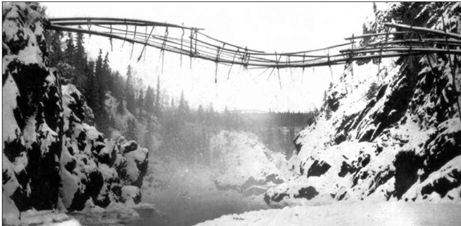
The first Hagwilget Bridge (1872) was built by the Hagwilget Indians using wooden poles tied together with cedar bark.
