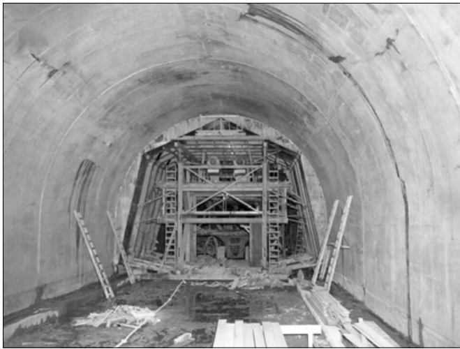
Trans-Canada Highway, Sailor Bar Tunnel concrete forms.
