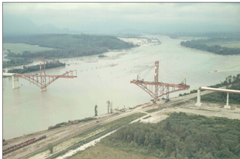
Port Mann Bridge, under construction.
