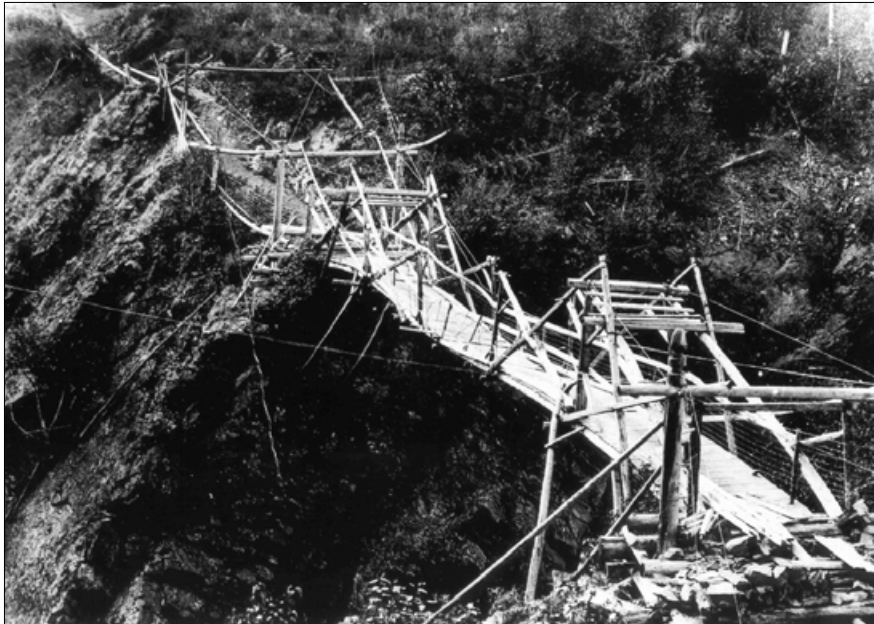
Second phase of the Hagwilget Bridge (1890s), reinforced with wooden poles and abandoned telegraph cable.
