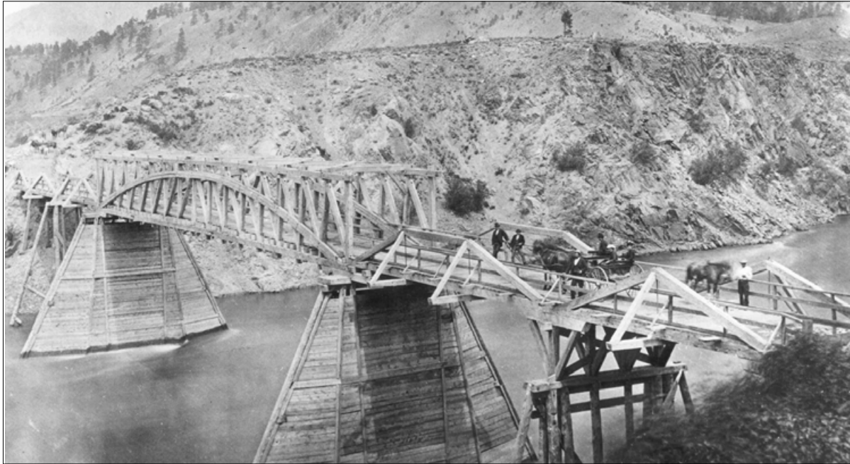
Bridges figured significantly in the early wagon roads. The elaborate truss bridge shown above was over the Thompson River. The suspension bridge built in 1863 was the first of three Alexandra Bridges to be built over the Fraser River, about 22.5 km north of Yale. The first bridge (shown below) was replaced in 1926 by a newer suspension bridge. The present steel arch span was completed in 1962.
