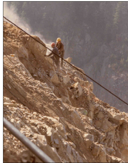
Hell's Gate Project, drilling for removal of fractured rock.
