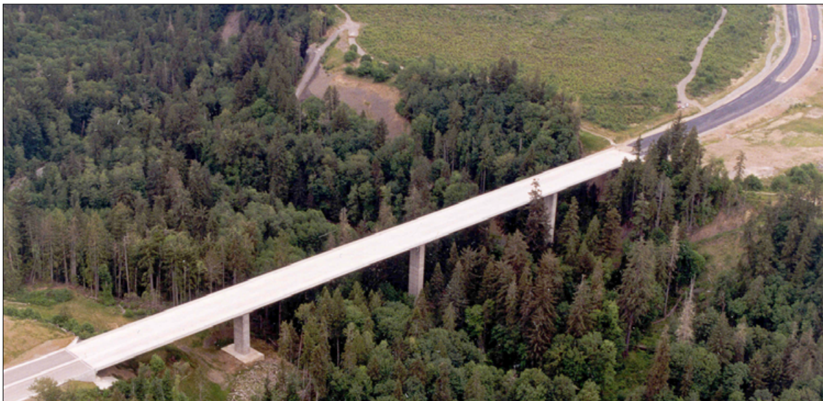
(Below) Tsable River Bridge.
