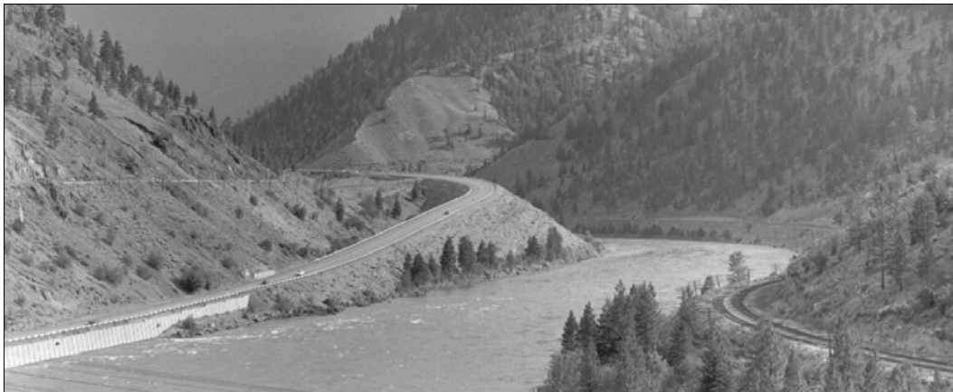
(Below) This section of the Trans-Canada Highway along the Thompson River swings out on high fill in order to maintain alignment and overpass the railway.
