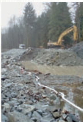
Pitt River – Landfill reclamation
