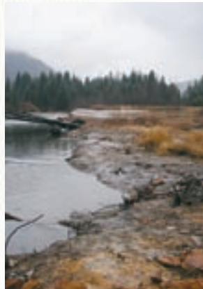
Yankee Girl tailings – Pre-erosion barrier construction
