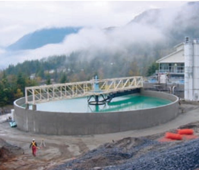
Britannia Mine water treatment plant under construction, Fall 2005
