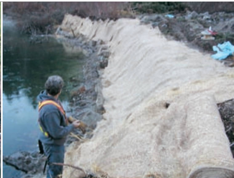
Malakwa – Installation of filter layer
