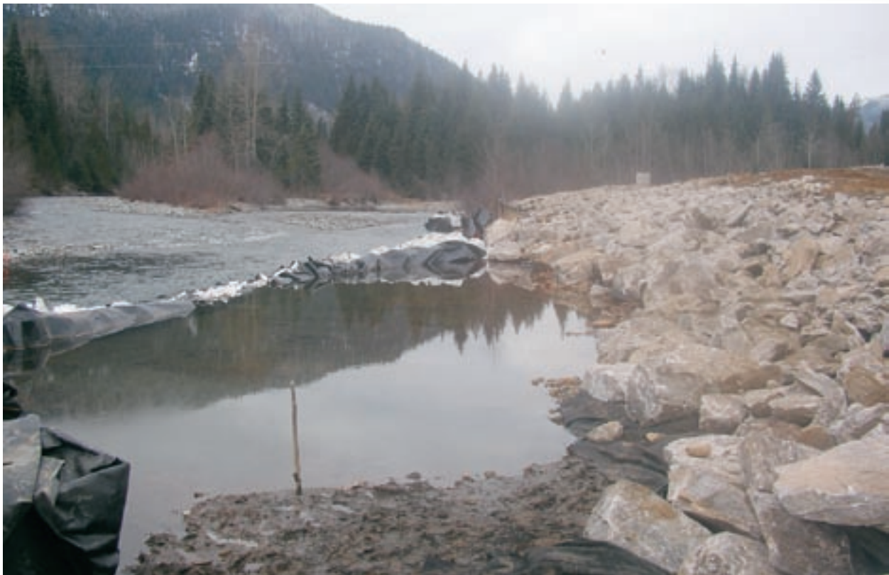
Yankee Girl tailings, Ymir – Erosion barrier adjacent to Salmo River
