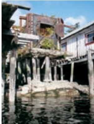
Goose Bay – Hazardous materials cleanup
