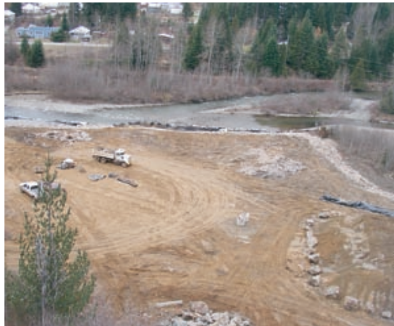
Yankee Girl – Erosion barrier construction, Fall 2005
