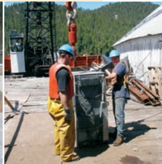
Goose Bay – Hazardous material removal
