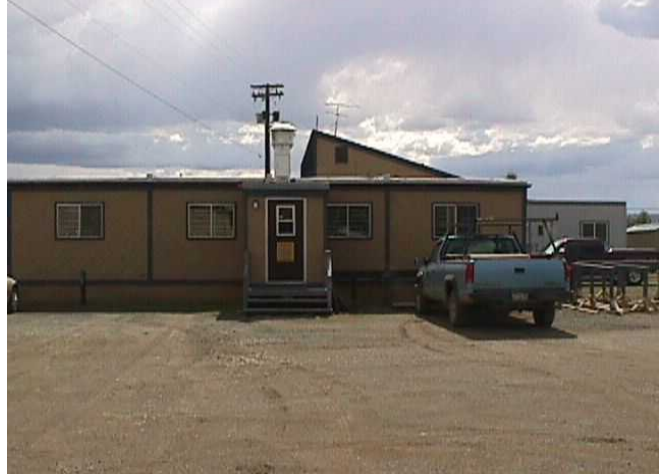
CNR site (Lakeland Mills) looking towards the south
