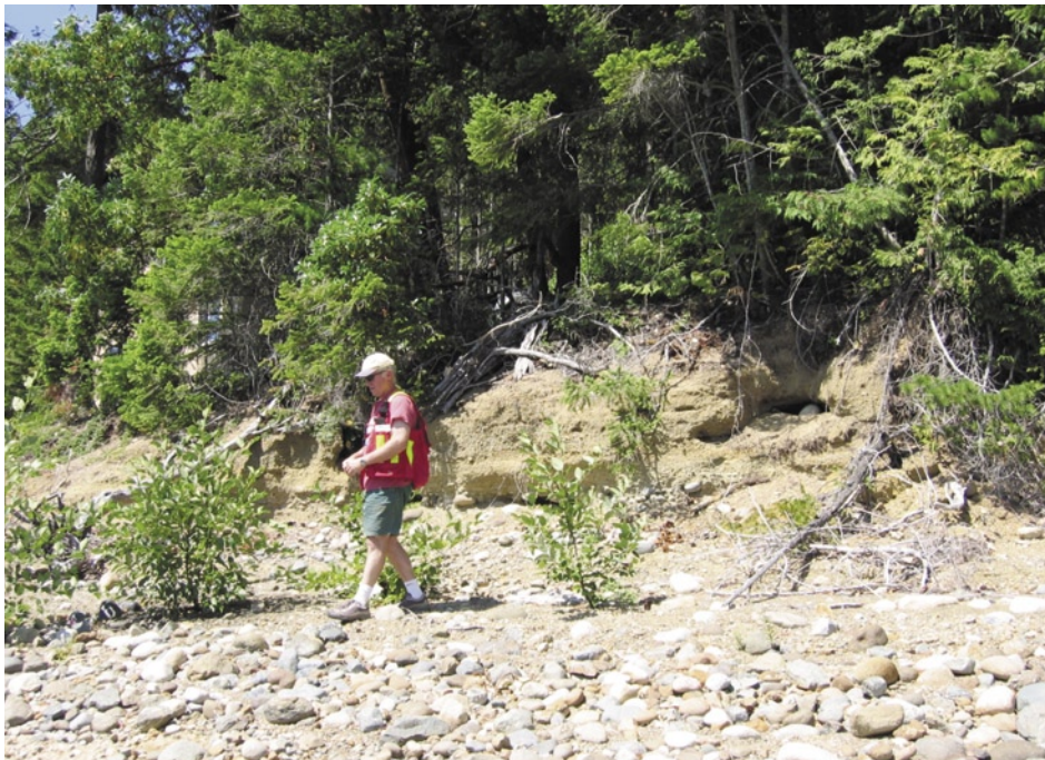
Figure 2. Exposed backshore is higher than 1 m. In this case, the sediment is non-cohesive but compact glaciofluvial sediments.
