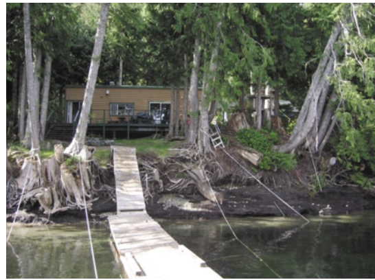
Figure 11. Profile and photographs showing the erosion hazard associated with vertical and exposed backshores consisting of non-cohesive material. Erosion hazard is related to bank height (and implicitly related to amount of potential loss of bank back from the shoreline). The photographs show two examples of Very High erosion hazards, where the bank is well in excess of 1 m high.
