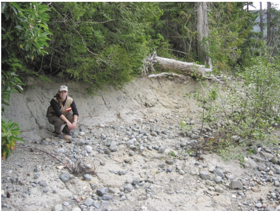
Figure 9. Profile and photograph of a beach with exposed but cemented banks. In this case the basal till remains exposed and resists vegetation, but it is also more resistant to erosion, and the erosion hazard is typically classed as Moderate.
