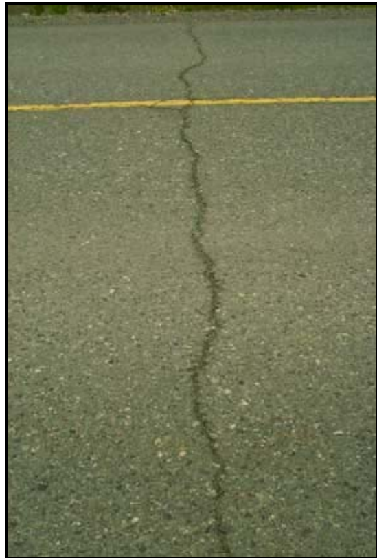
Figure 14 - Moderate Severity TC
