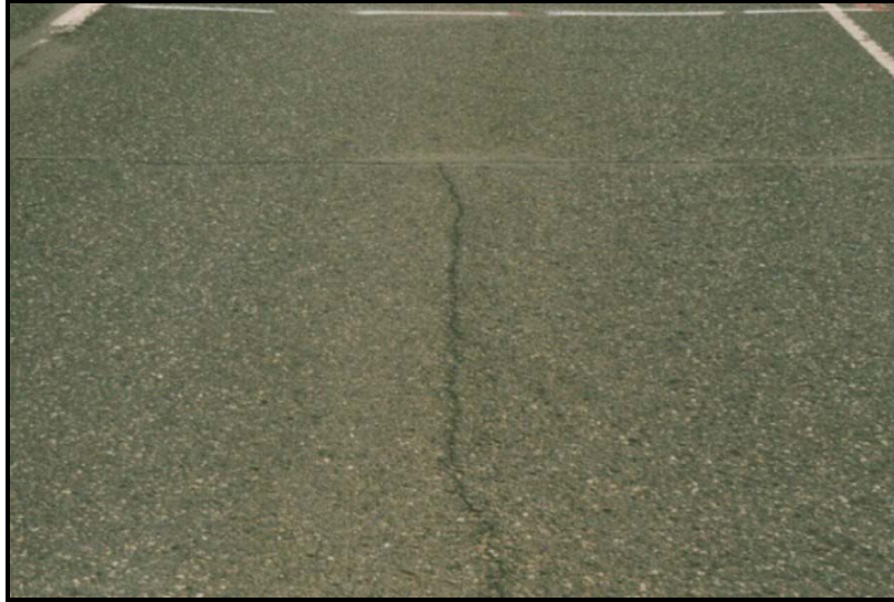
Figure 17- Low Severity MLC
