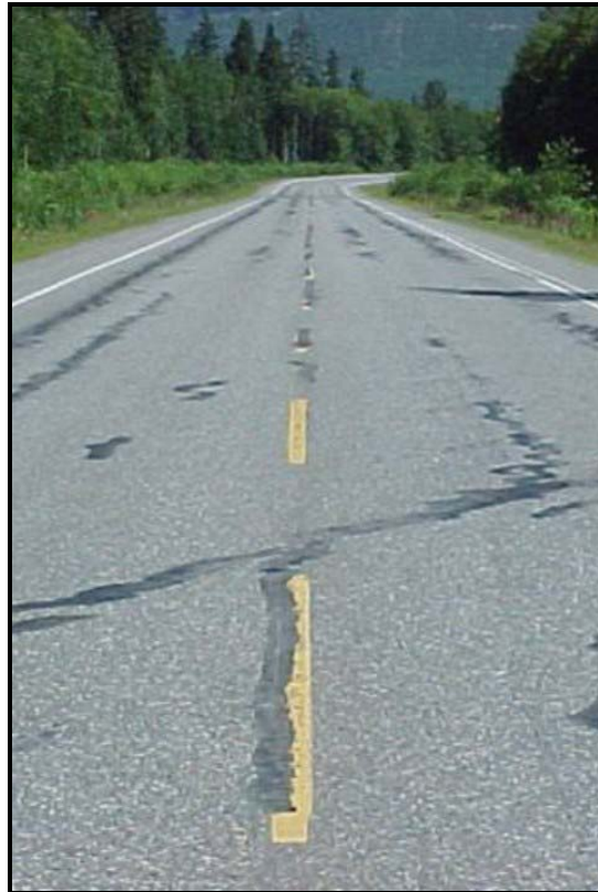
Figure 44 - Level 3 Sealing
