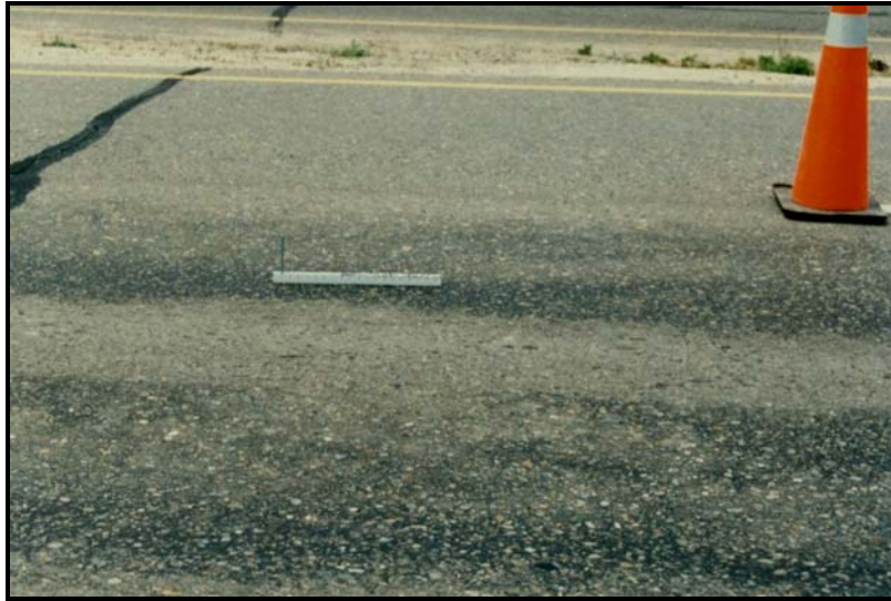
Figure 33 - Moderate Severity BLD
