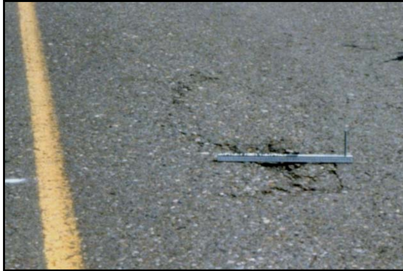
Figure 35 - Low Severity POT
