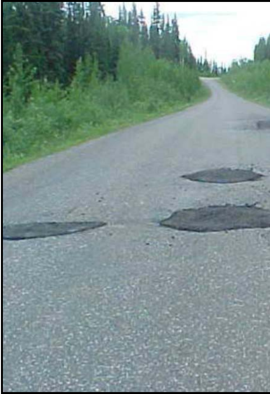
Figure 45 - Level 1 Patching
