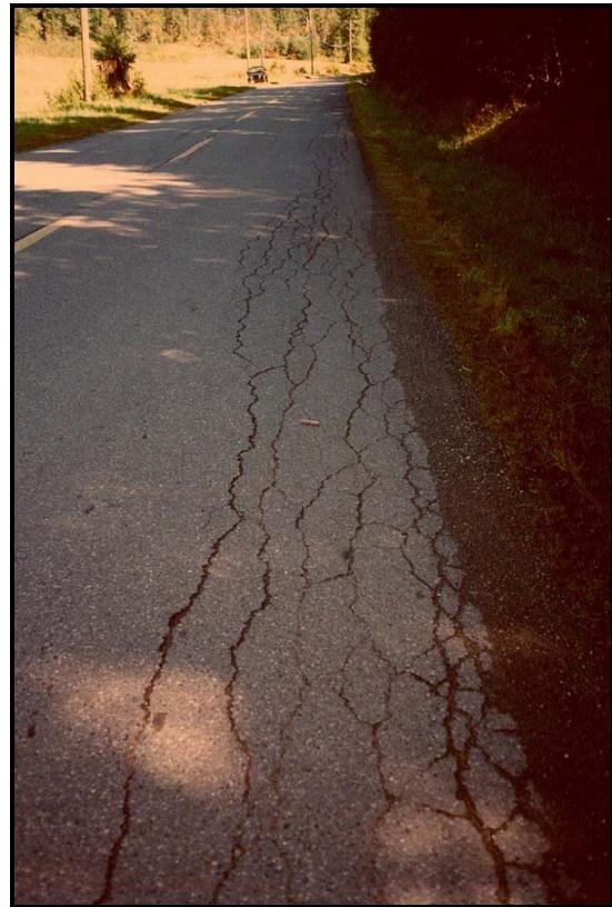
Figure 12 - High Severity PEC
