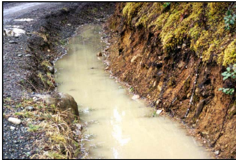
Figure 42 – Unacceptable Drainage
