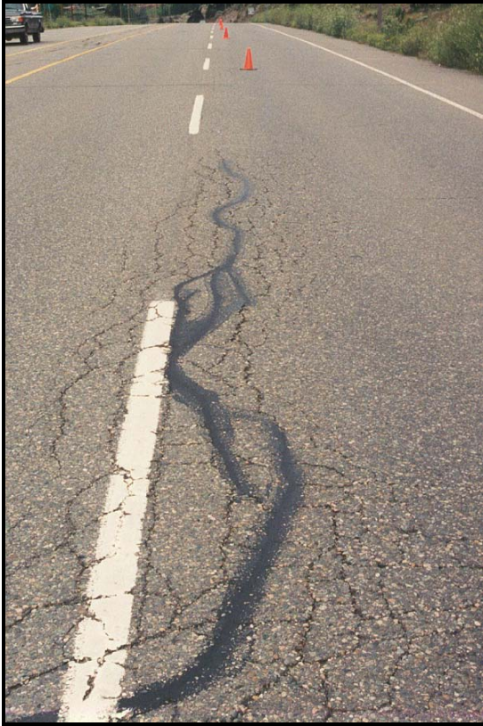
Figure 43 - Level 1 Sealing
