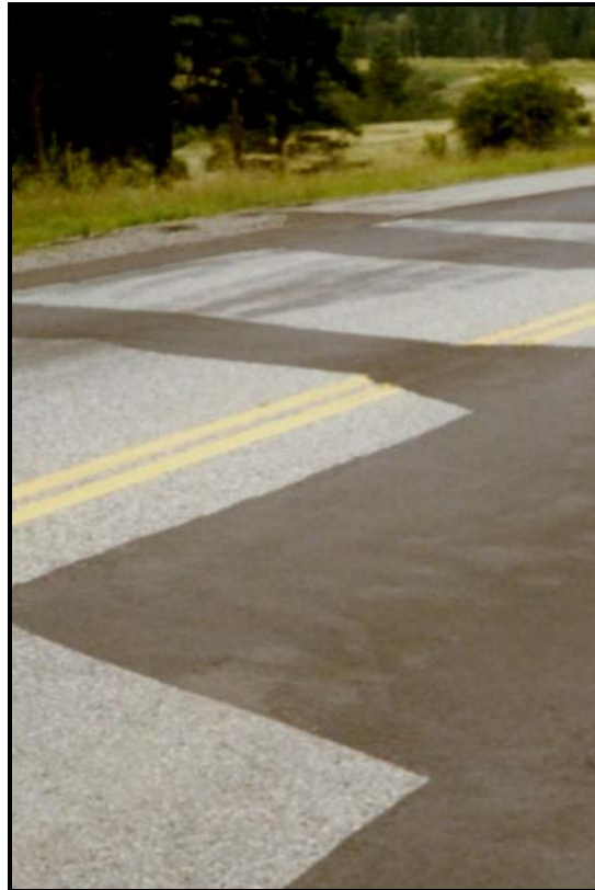
Figure 46 - Level 2 Patching
