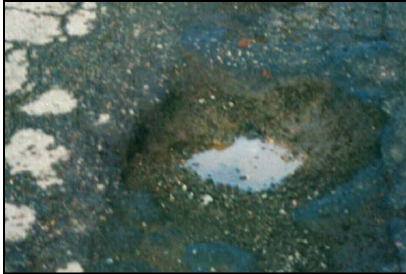
Figure 37 - High Severity POT
