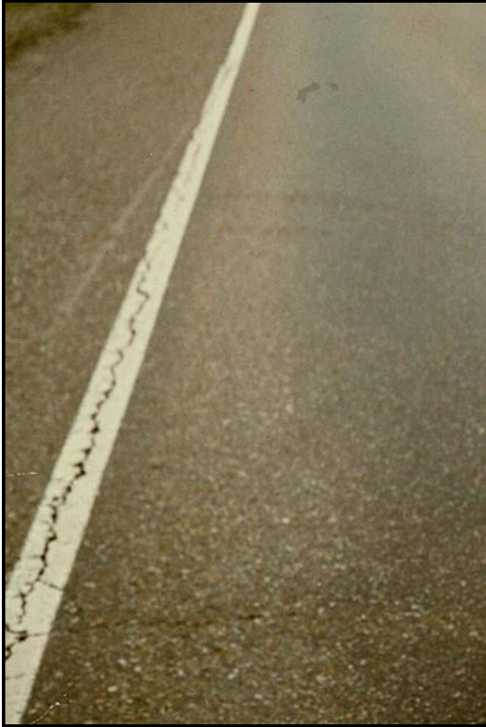
Figure 9 - Low Severity PEC
