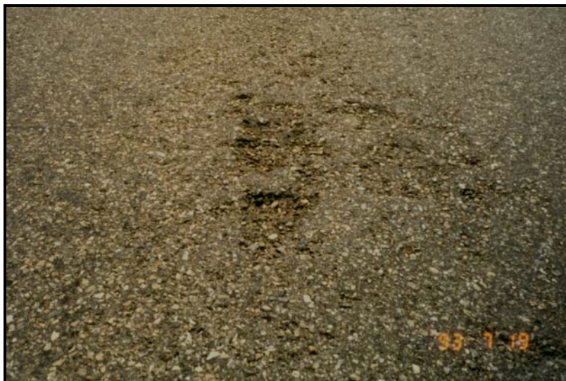
Figure 40 - High Severity RAV
