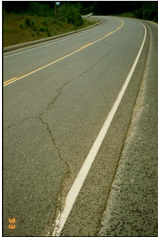
Figure 20 - High Severity MLC
