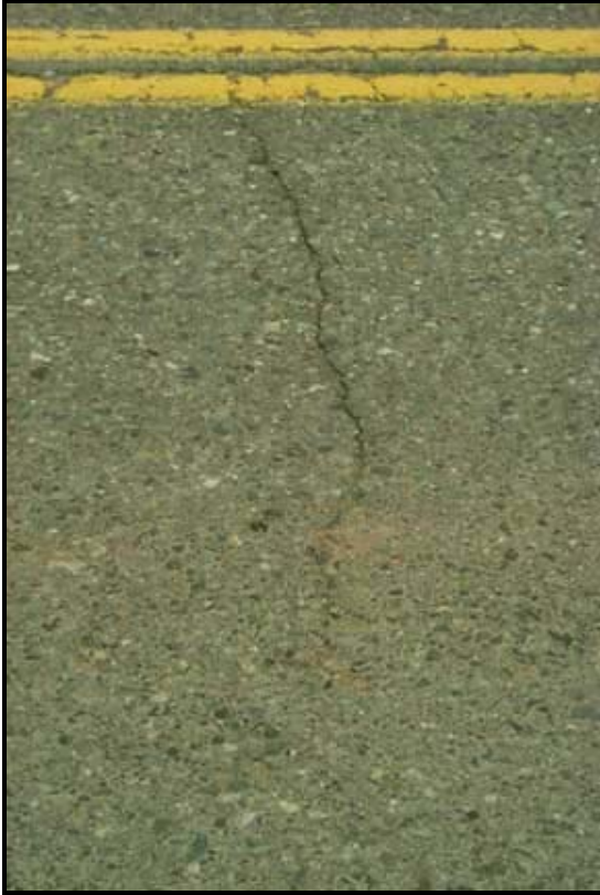
Figure 13 - Low Severity TC
