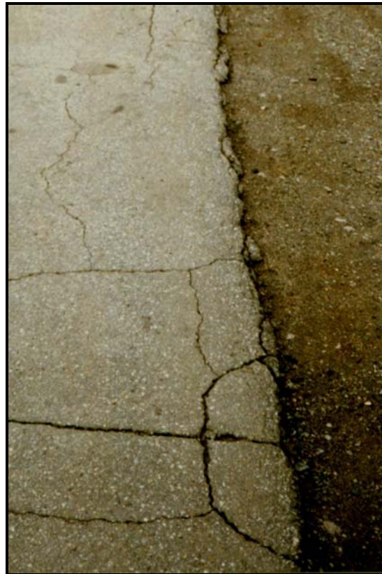
Figure 10 - Moderate Severity PEC
