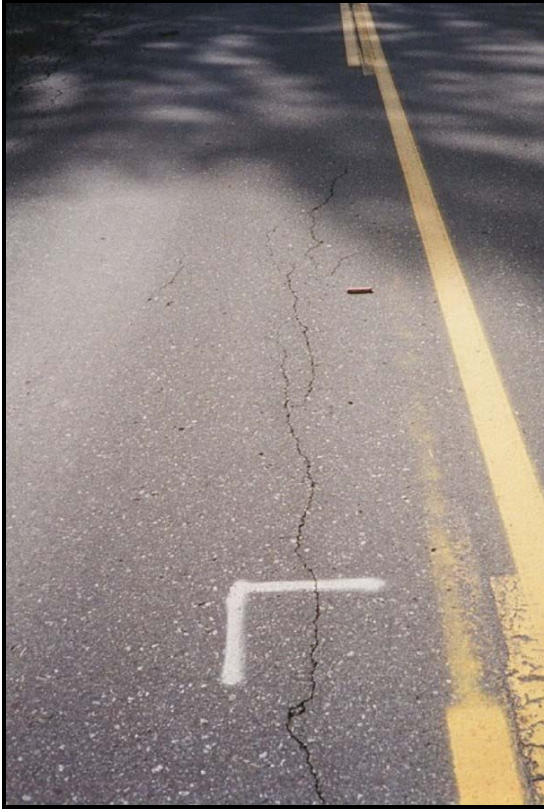
Figure 1 - Low Severity LWP
