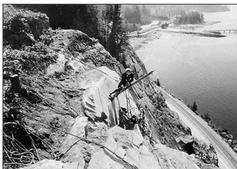
Implementing safety improvements: Rock bolt installation
