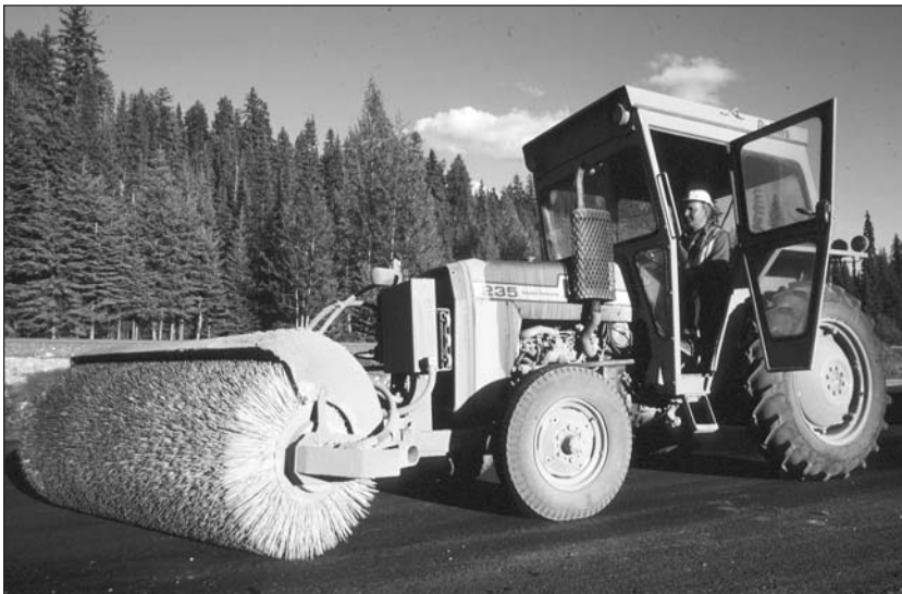
Road widening construction north of Prince George
