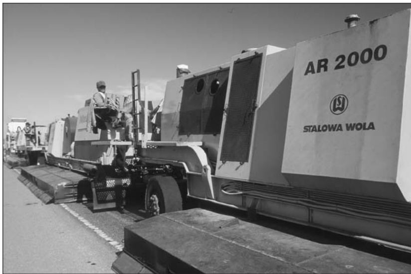
Rehabilitating the highways: Fresh asphalt re-paving
