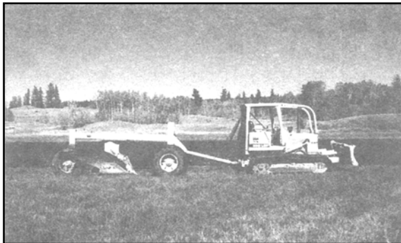
Figure 9. BCMAFF flow and low ground pressure crawler
