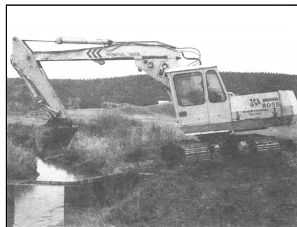
Figure 6. Track-type hydraulic excavator.
