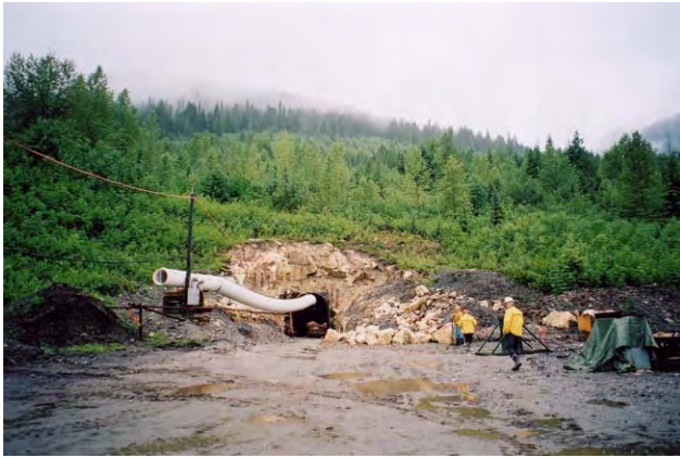
Photo 8. Portal area at the MAX molybdenum site being readied for production in late 2006.
