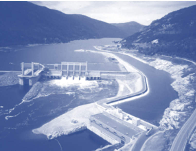
Arrow Lakes Generating Station
