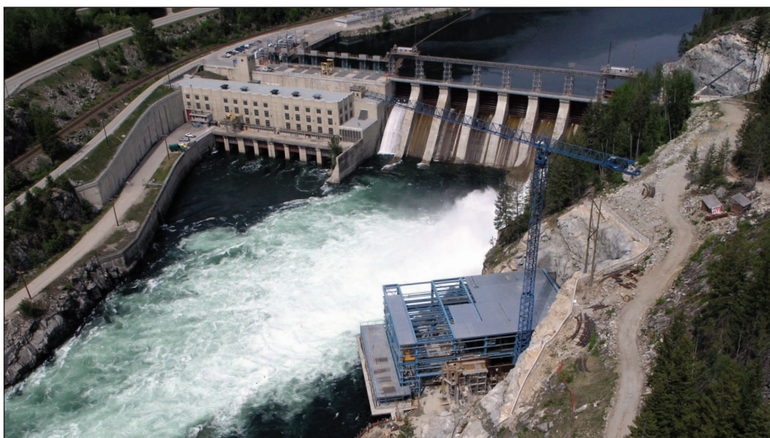
Brilliant dam and Brilliant Expansion (under construction)
