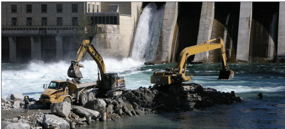
Removing the berm at Brilliant Expansion
