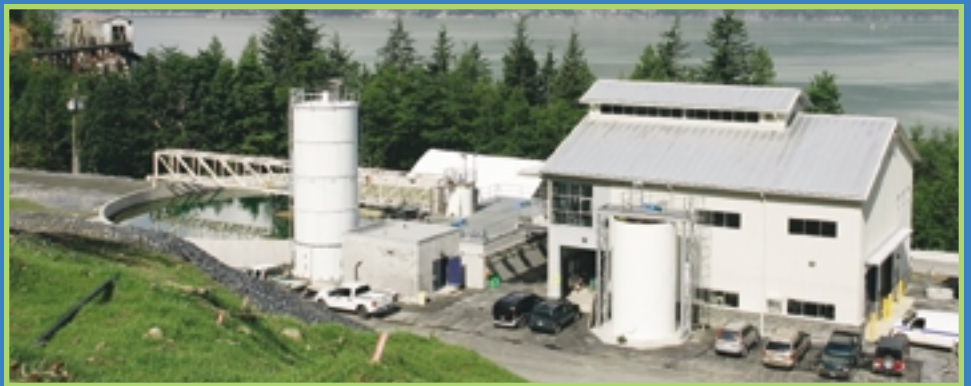
Britannia Mine Water Treatment Plant
