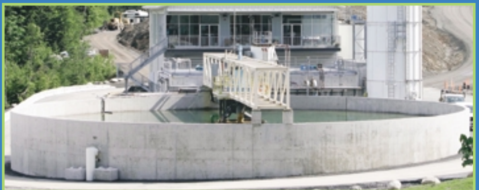
Britannia Mine Water Treatment Plant
