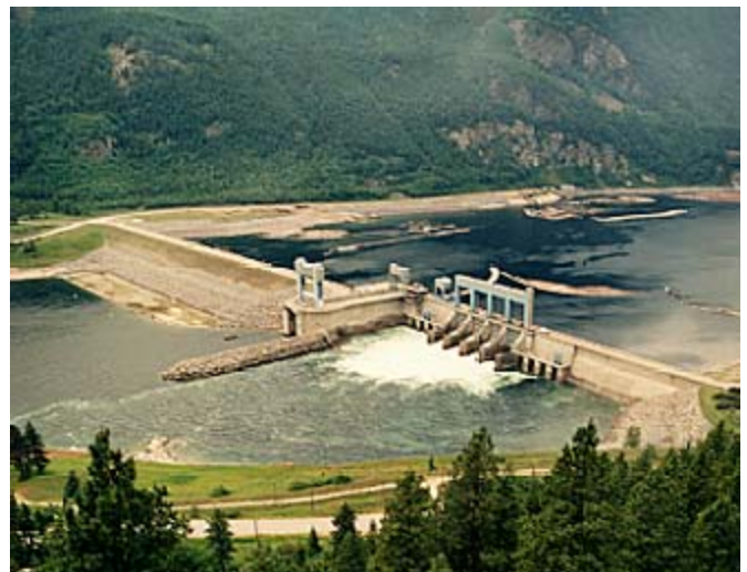
Hugh Keenleyside Dam is an earthfill and concrete structure that incorporates a navigation lock, four spillways, and eight low-level ports. A remediation project, planned for completion in 2011, will mitigate earthquake risk and protect public safety.
