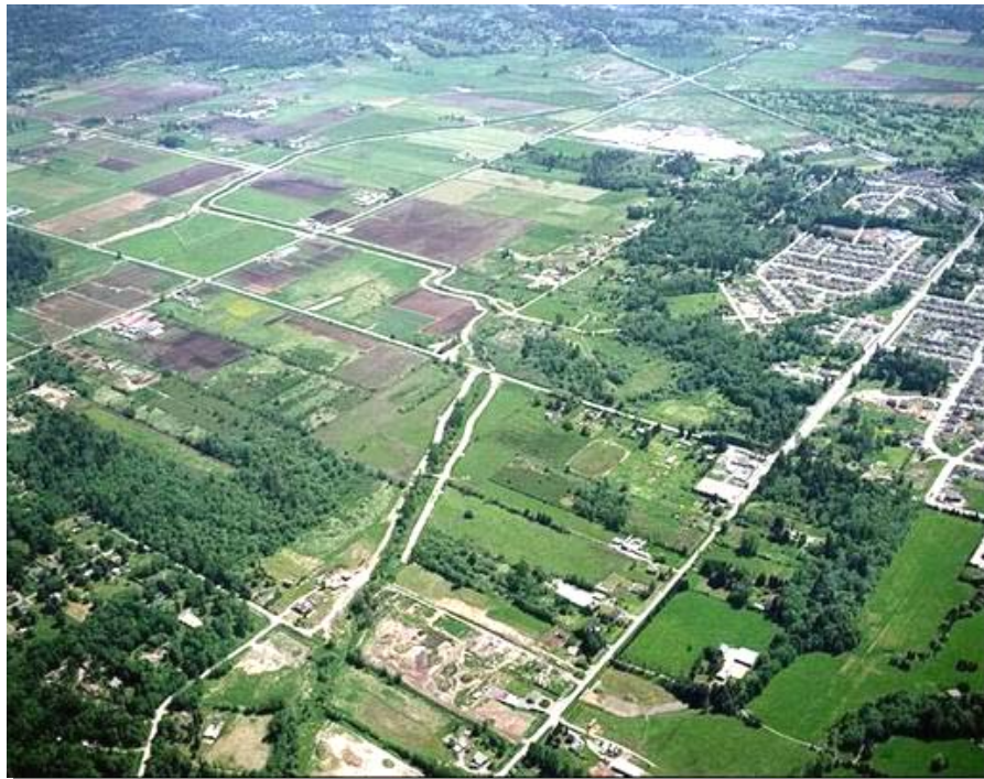
Upper Serpentine Dyke Tie-In October 2001
