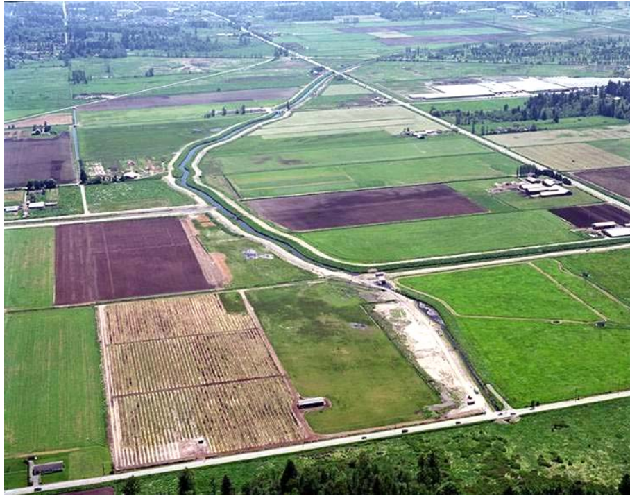
Upper Serpentine Pump Station – April 2001
