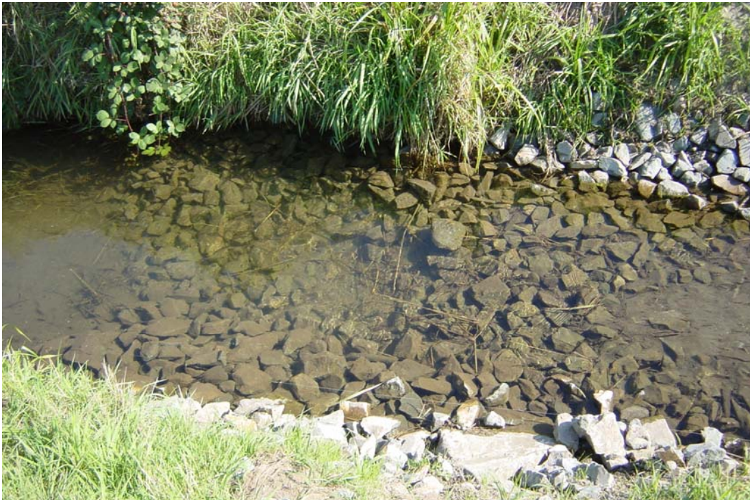
Figure 21. Example of Rock-weir structure installed in Big Ditch.
