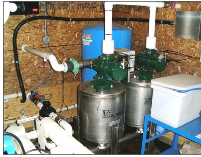
Figure 2 Sand Filter Units
