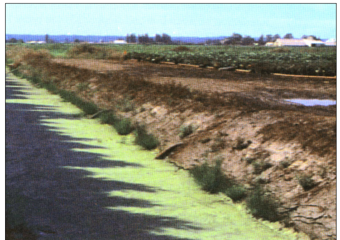
Figure 1 Drainage Ditch Used for Irrigation Supply
