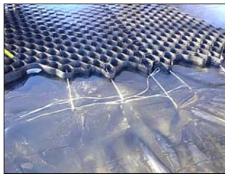
Geocell Laid On Top
