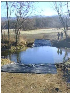
Geotextile Laid
