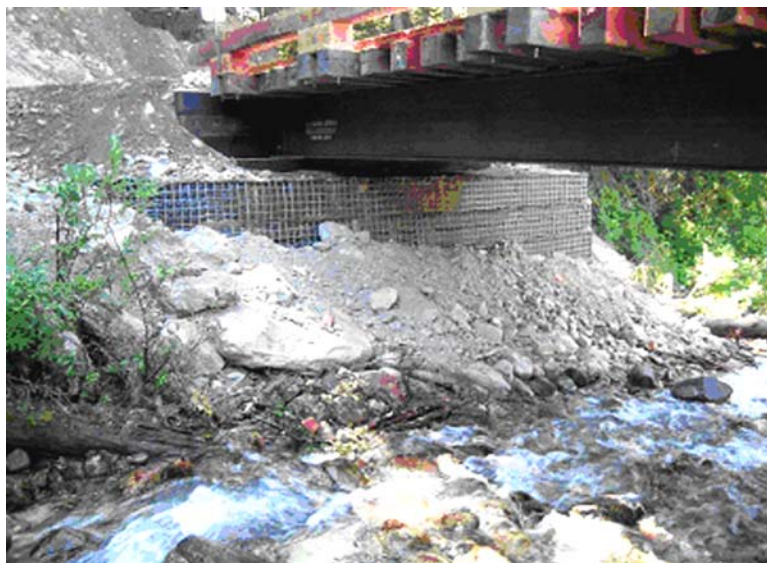
Figure 6 A Reinforced Soil Bridge Abutment
