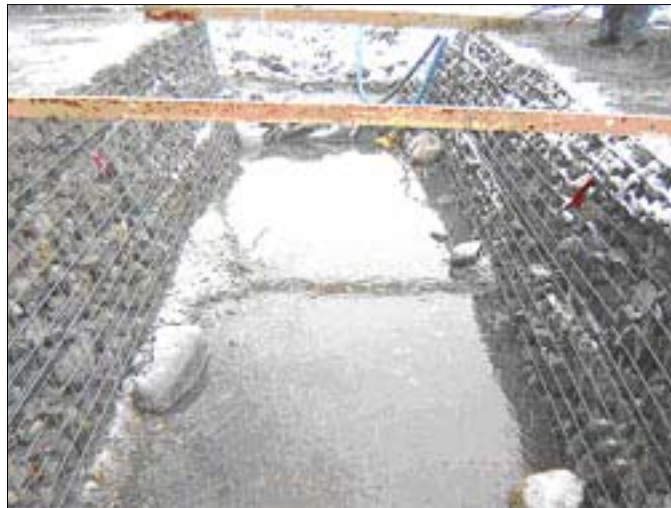
THE REINFORCED SOIL ABUTMENTS ARE READY FOR THE STRINGER INSTALLATION
