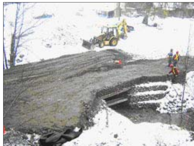
Figure 7 Basic Construction Steps for a Reinforced Soil Stream Crossing
