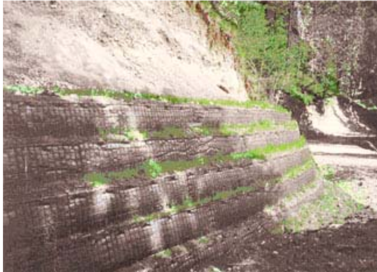
Figure 5 A Reinforced Soil Retaining Wall
