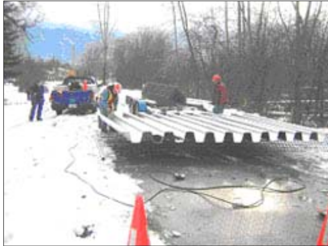
THE FORMED SHEET STEEL STRINGER IS ASSEMBLED
