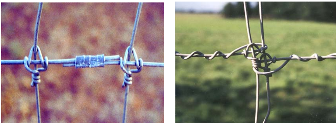
Figure 7 Woven Wire Connections: Nicopress sleeves (left) and Twist Wrap Knot (right)
