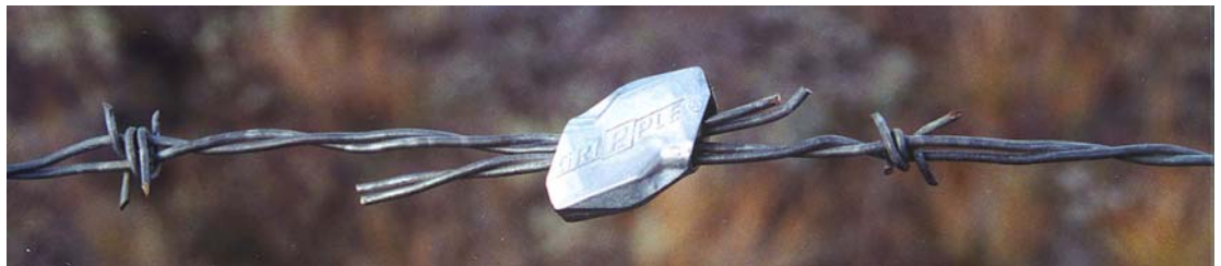
Figure 4 Knots and Mechanical Splice for Barbed Wire
