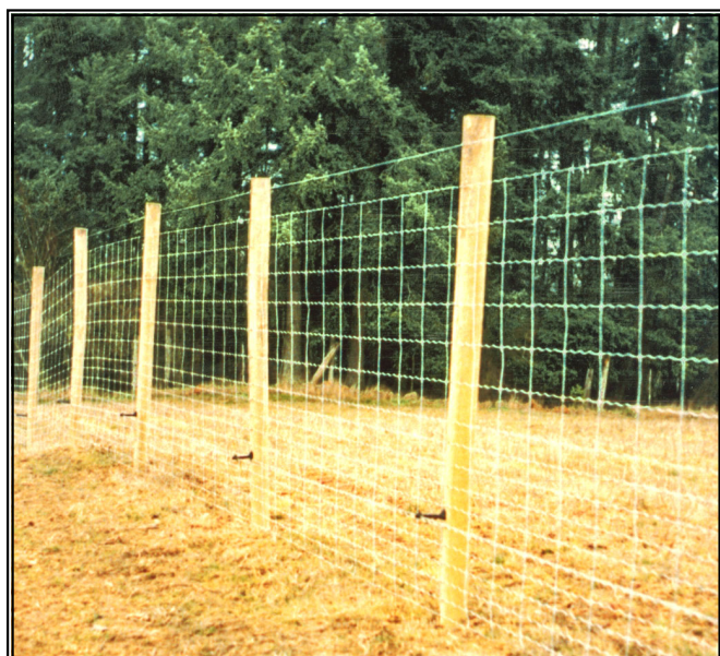
Figure 1 Typical Deer Exclusion Fence
