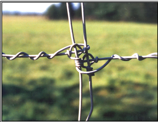
Figure 4 Splicing Woven Wire
