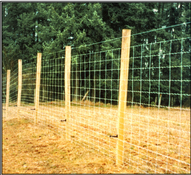
Figure 1 Typical Elk Exclusion Fence Using Woven Wire
