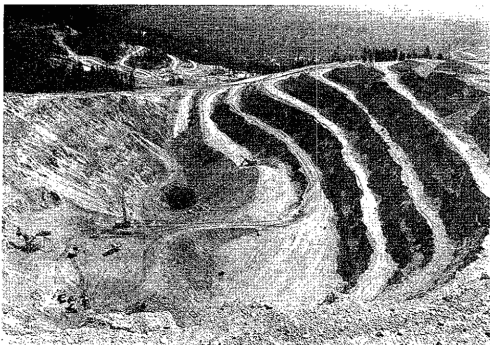
Craigmont open pit, August, 1963. The final benches are 66 feet high.
