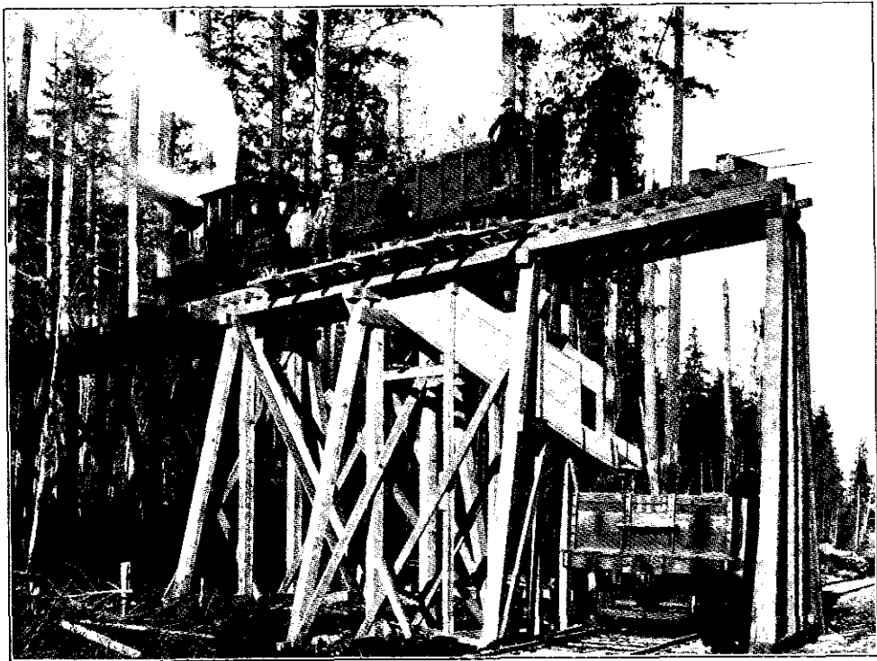
LENORA MINE—STEAM TRAMWAY CONNECTING WITH E. & N. RY.
