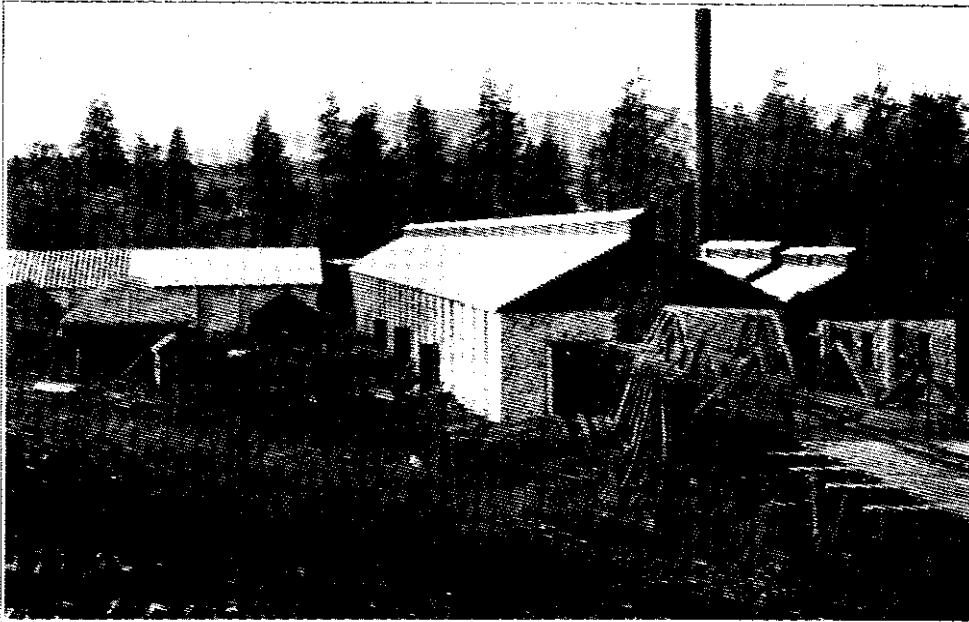
Cement-works under Construction at East Princeton.
