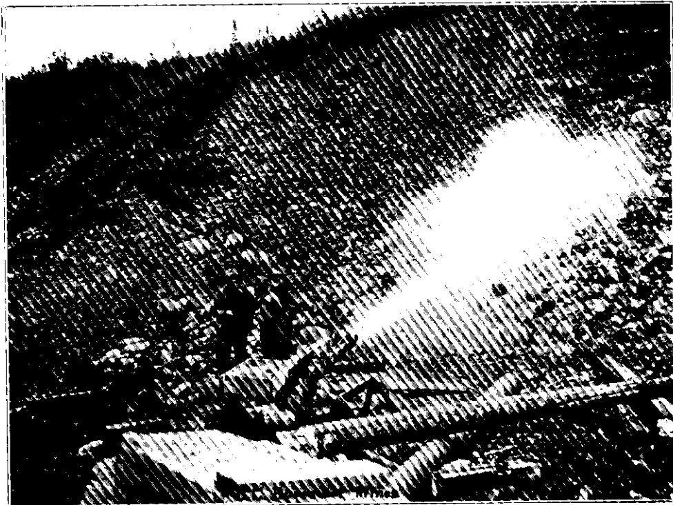
Opening Hydraulic Pit, Boulder Creek Mining Co.
