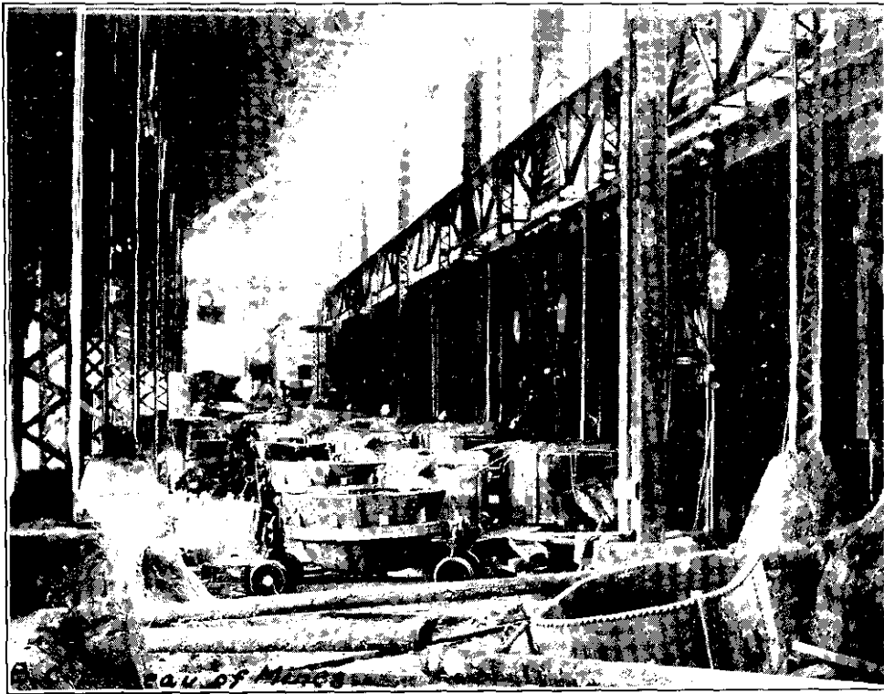
Furnace-shed, Granby Smelter, Grand Forks.
