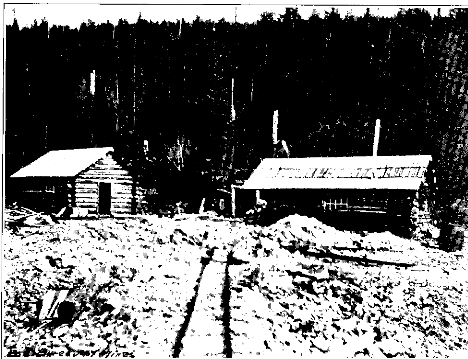
Lower Tunnel, Bayonne Mine—Nelson M.D.
