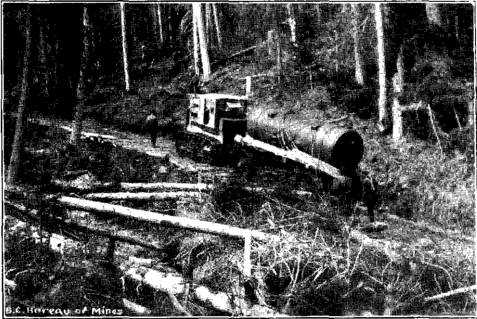
Henderson Mine—Tractor transporting Boiler.
