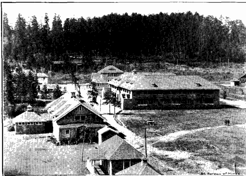
Cassidy Colliery, Granby C.M.S. & P. Co.—Rooming-house.
