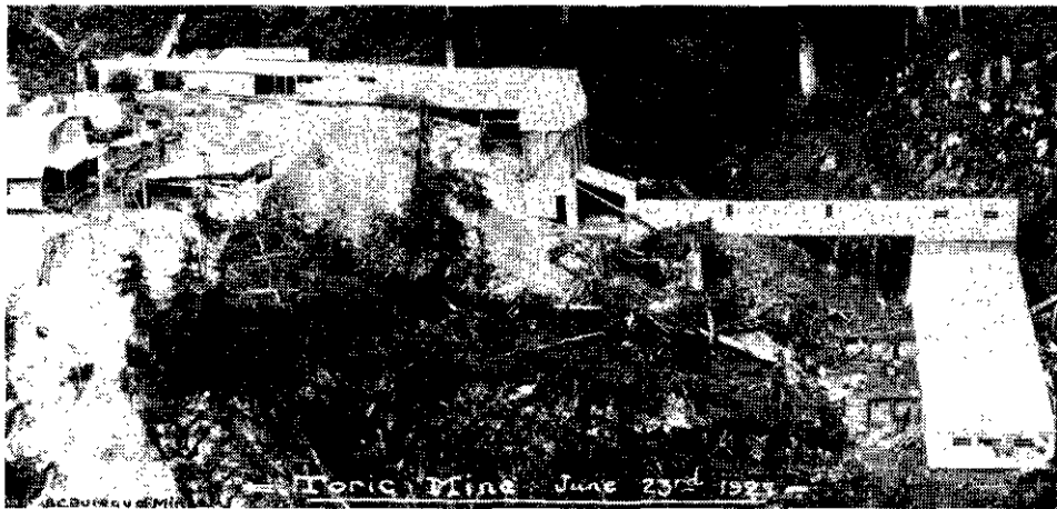
Toric Mines, Ltd.—Mine Plant.
