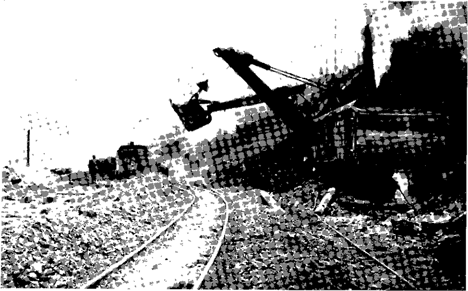
Corbin Colliery—Stripping No. 5.
