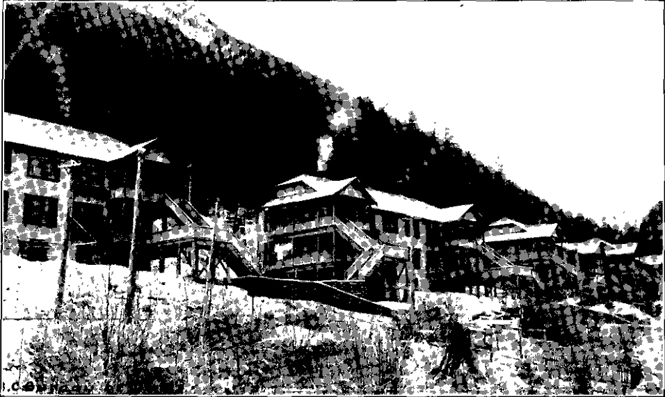
Britannia Mining and Smelting Co.—Upper Camp, Vancouver M.D.
