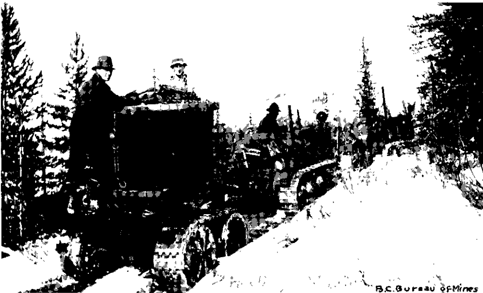
Reno Gold Mines, Ltd.—Taking up Aerial Tram Cable.
