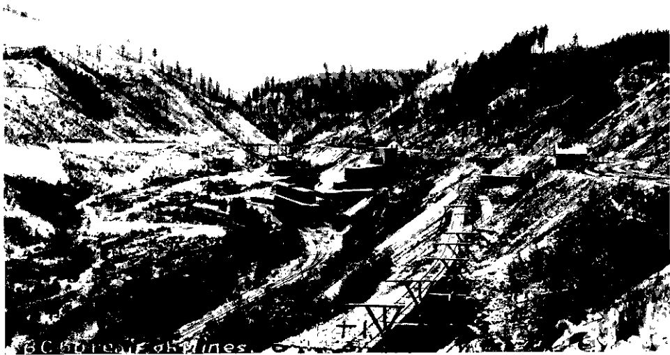
Sullivan Mine—Crushers at Portal of Main Tunnel.
