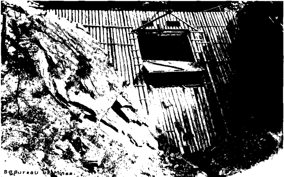
Weaver Creek—A Boomer Gate for Placer-mining.
