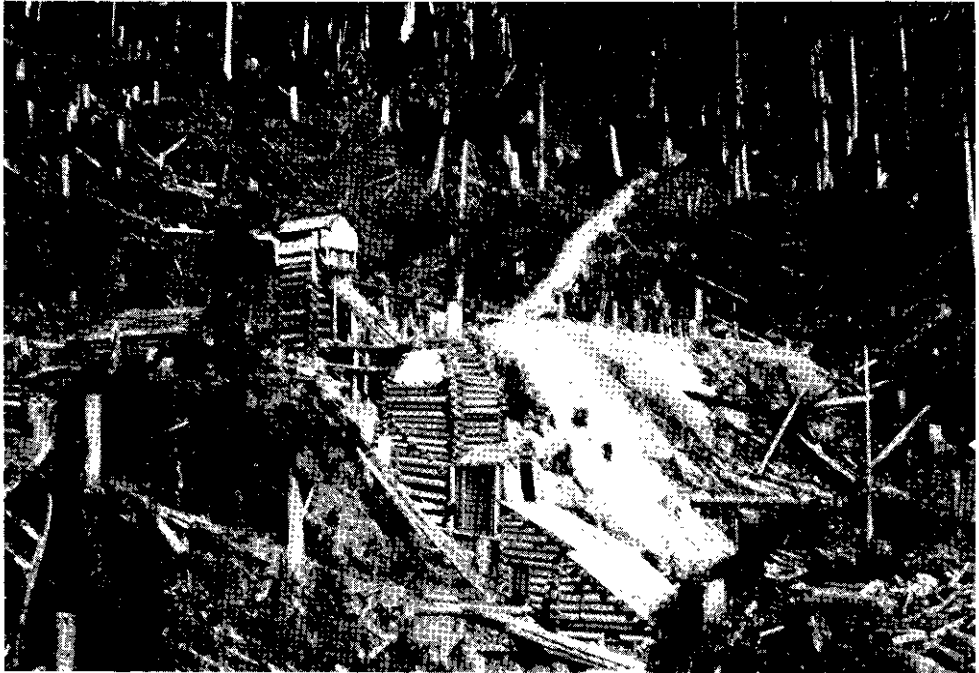
Home Gold Mining Co., Ltd. Mill, Coquitalla Area.
