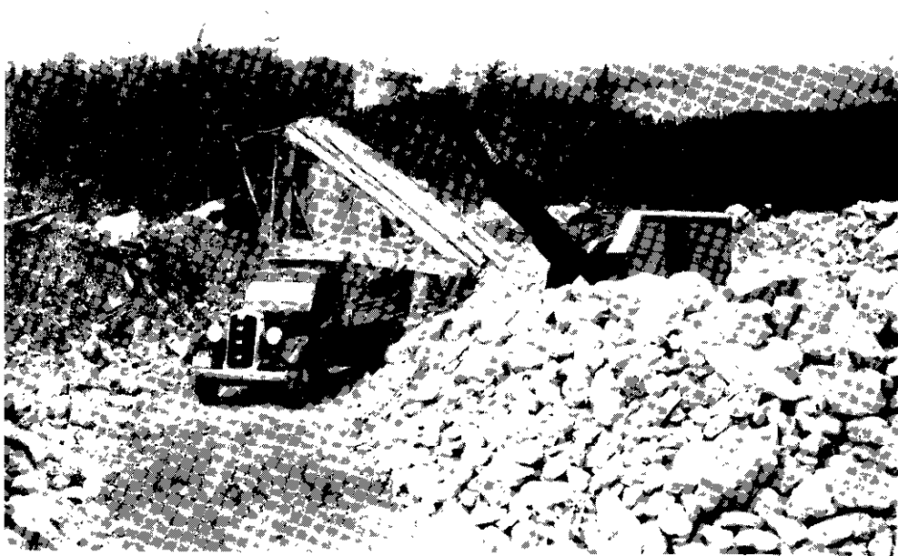
Powershovel, loading-pocket, and truck, Inca Placer Pit, Palmer Bar Creek.
